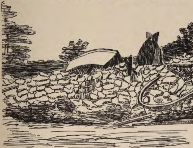
FIG. 2.—Ruins of a stone church after the Indian earthquake of June 12, 1897 (after R. D. Oldham).
